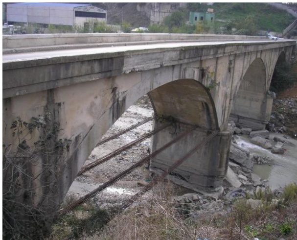
Figure 1 Beshiri Bridge- Longitudinal view
